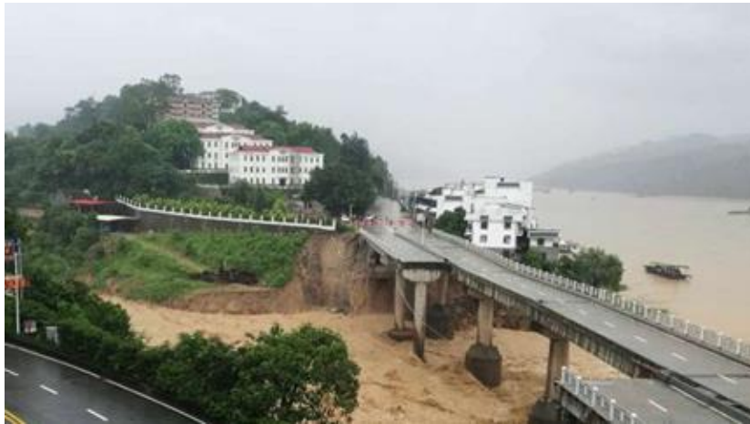
Figure 1: Collapsed fly-over in Minqing county
