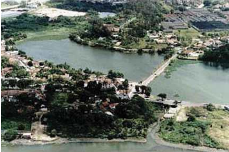
Figure 1 - Weir of Apipucos - the oldest dam in Brazil
